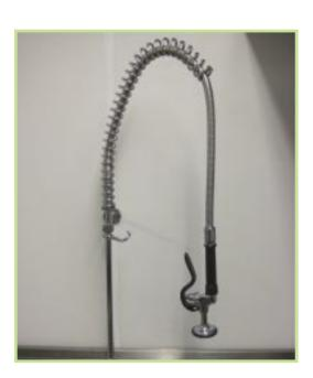
In your kitchen install low flow trigger operated spray taps and hoses.
