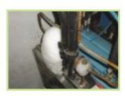
A poorly maintained beer chilling system. Ice build up indicates poorly insulated pipework on refrigeration.
