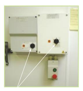
Variable speed drives can reduce energy consumption for extractor fans
