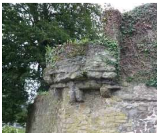
Fig 17 Detail of the Bartizan to north east junction of Town Wall
