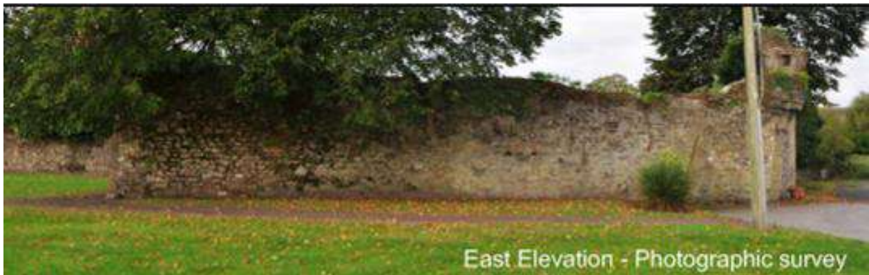
Fig 16 Panorama view in internal Wall at tennis court and east elevation at Castle Park
