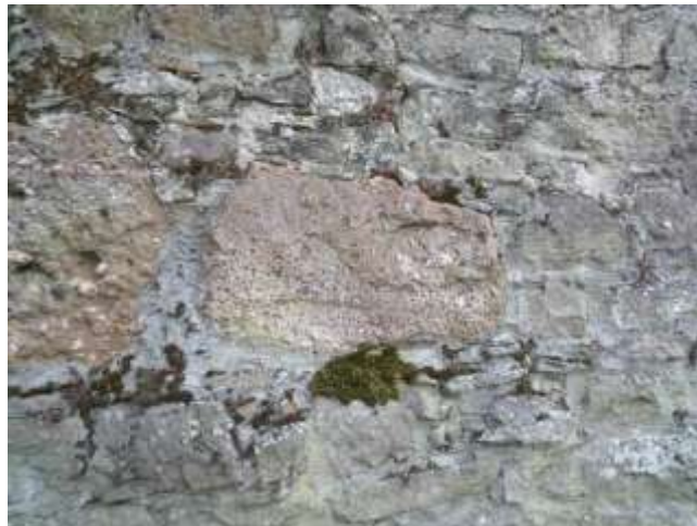
Fig 18 Detail to right showing variety of stone including conglomerate stone (individual stone within the matrix of the rock) which can also be seen in the retaining wall to St Molleran's Church in Carrickbeg.
