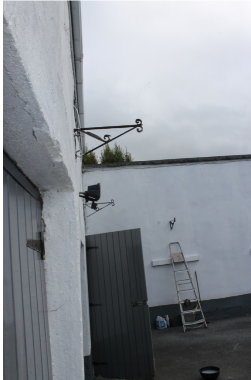
Area 1 – Front Wall of Adjoining Storage Building – Taken 24/10/14
