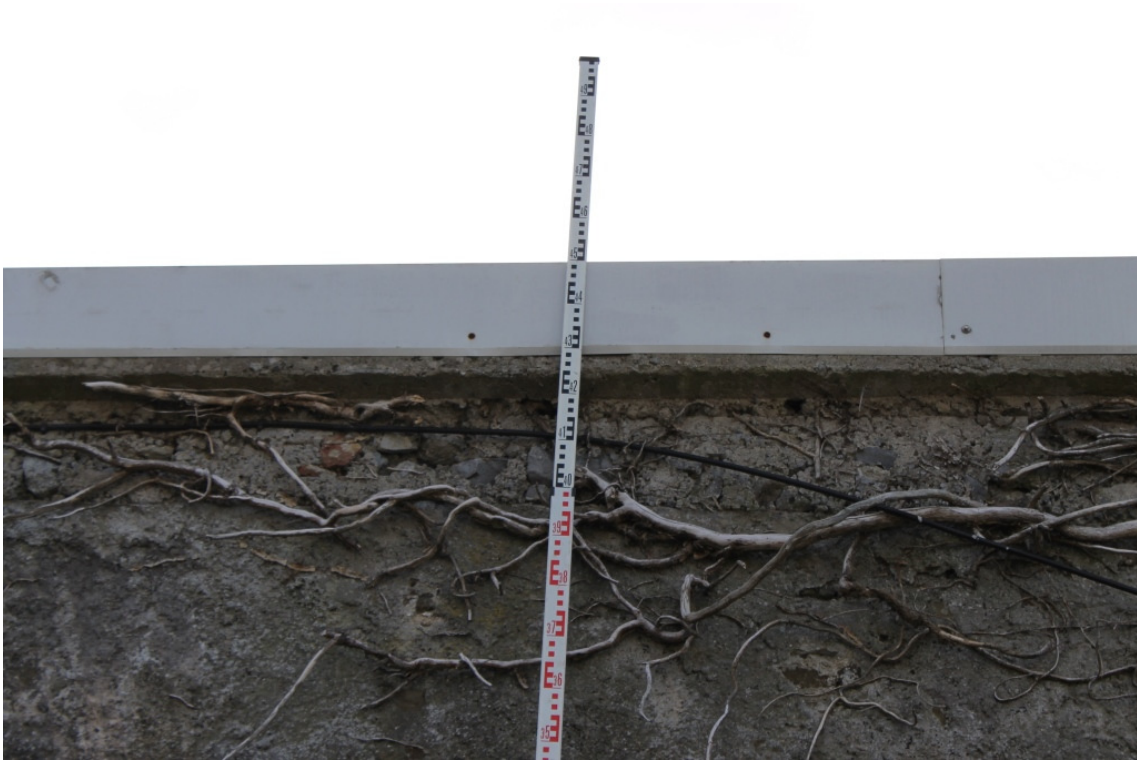
Area 1 – External Face – Note Concrete Capping and Metal Fascia - Taken 24/10/14
