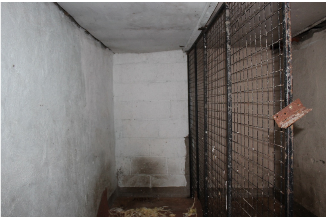
Area 1 - Internal Face – Note Internal block Wall – Taken 24/10/14
