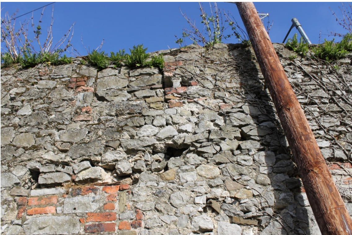
Area 2 – Internal Face – Note Filled Openings and Timber Lintel - Taken 24/10/14
