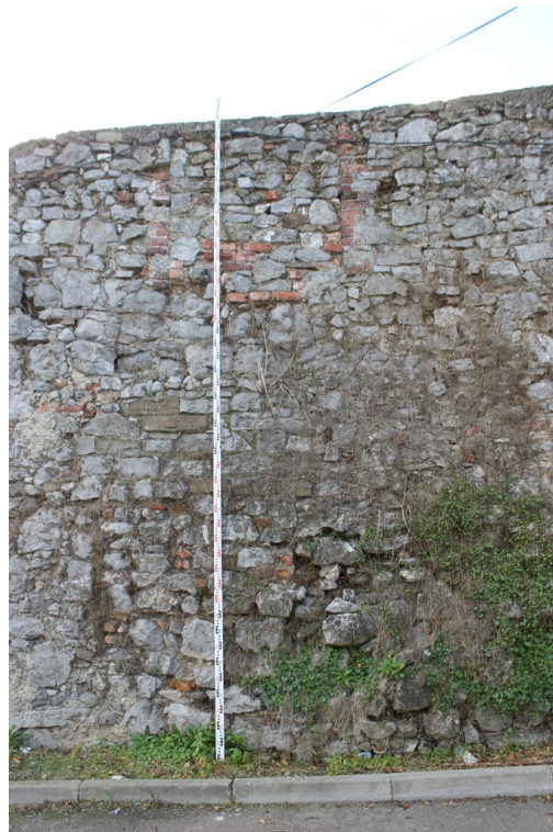
Area 2 – External Face - Taken 24/10/14
