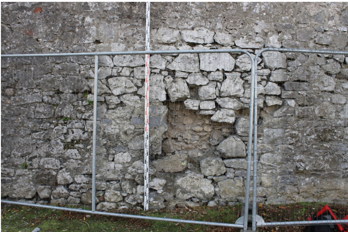
Area 1 – External Face – Taken 24/10/14
