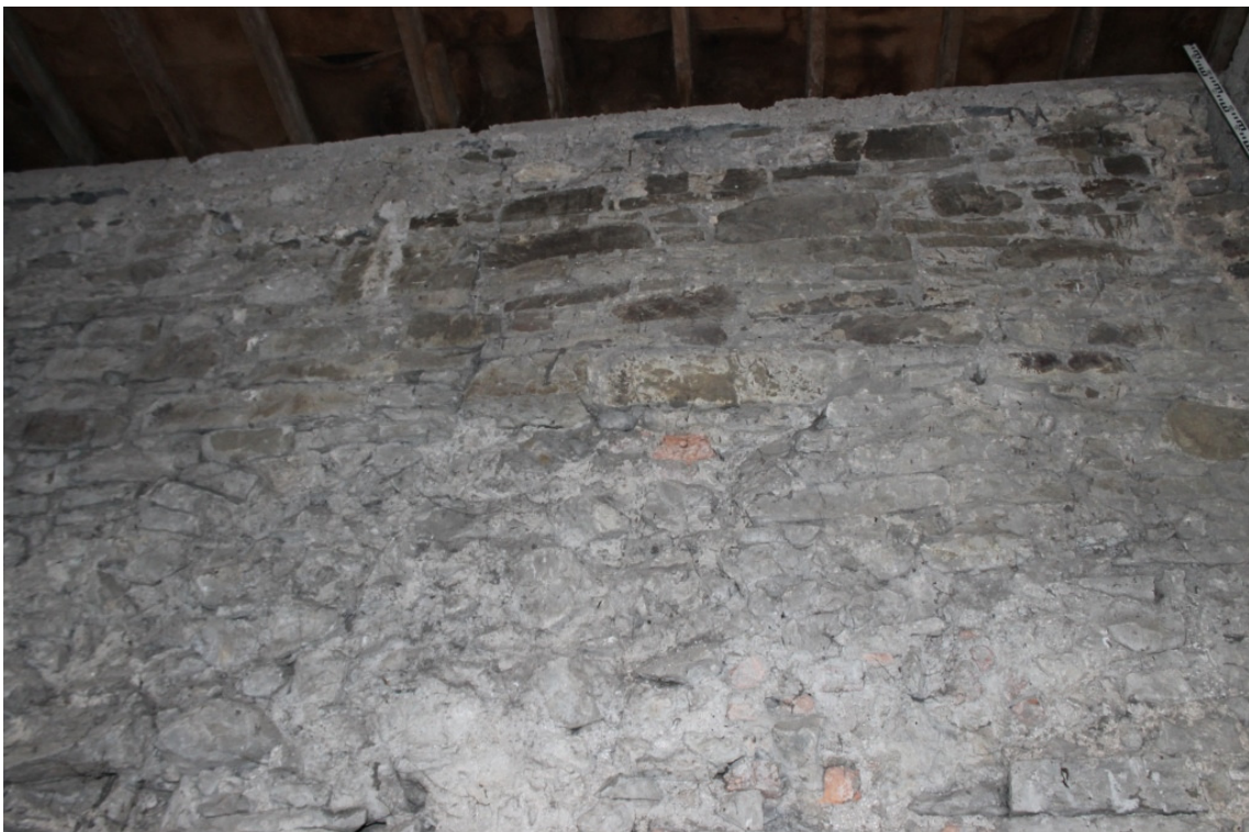
Area 1 – Internal face – Change of Stone – Taken 24/10/14
