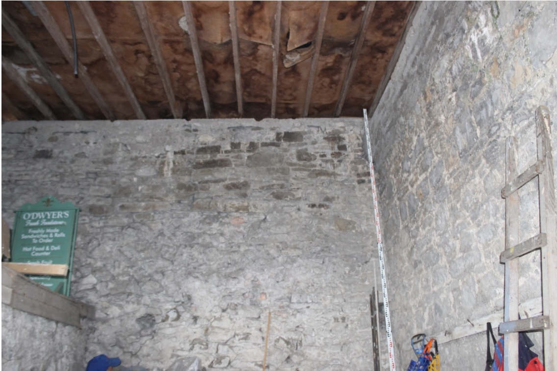
Area 1 – Internal Face – Taken 24/10/14
