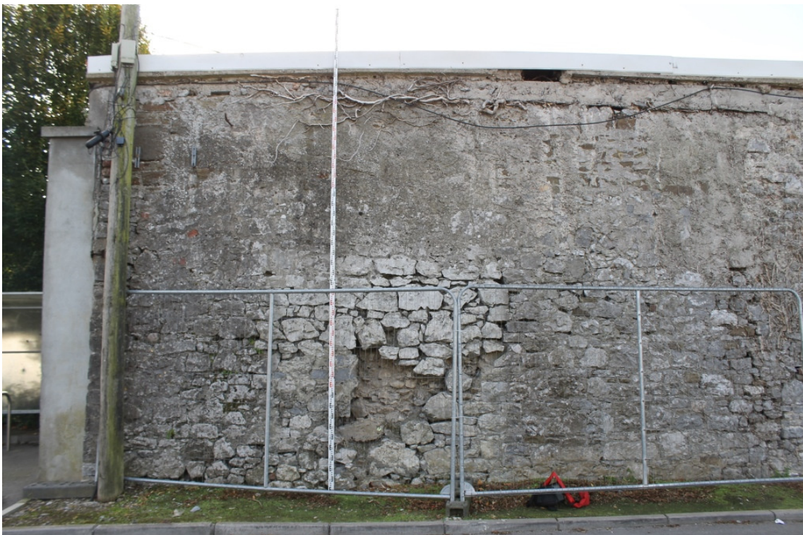
Area 1 – External Face – Taken 24/10/14
