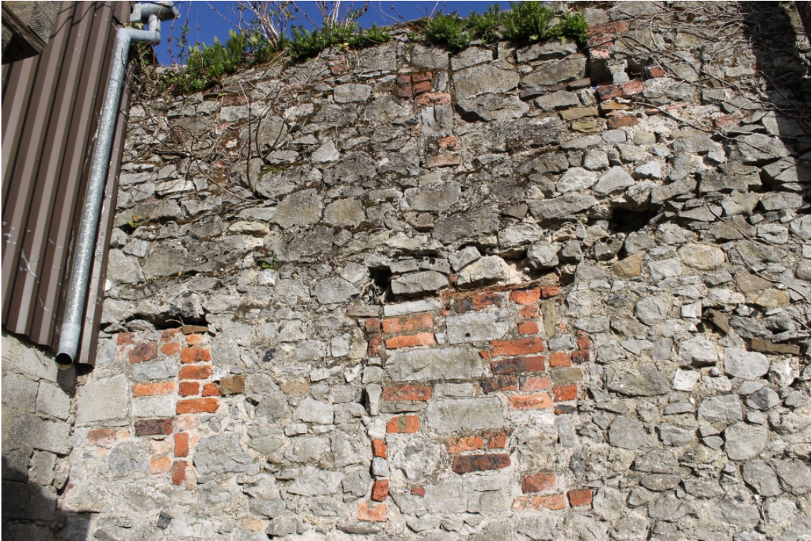
Area 2 – Internal Face – Note Filled Openings and Downpipe - Taken 24/10/14
