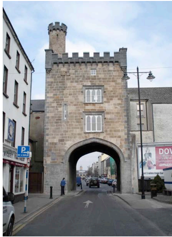
West gate from west
