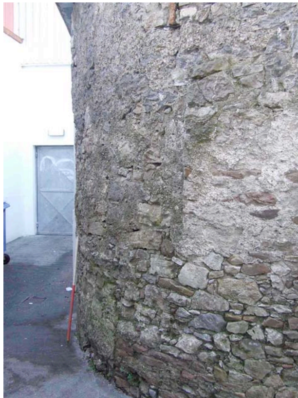
North-east corner turret incorporated into modern development
