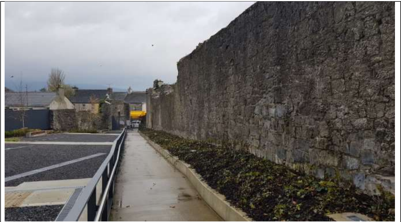
i. East face of Town Wall (facing into new public park), following completion of works – 7/11/19
