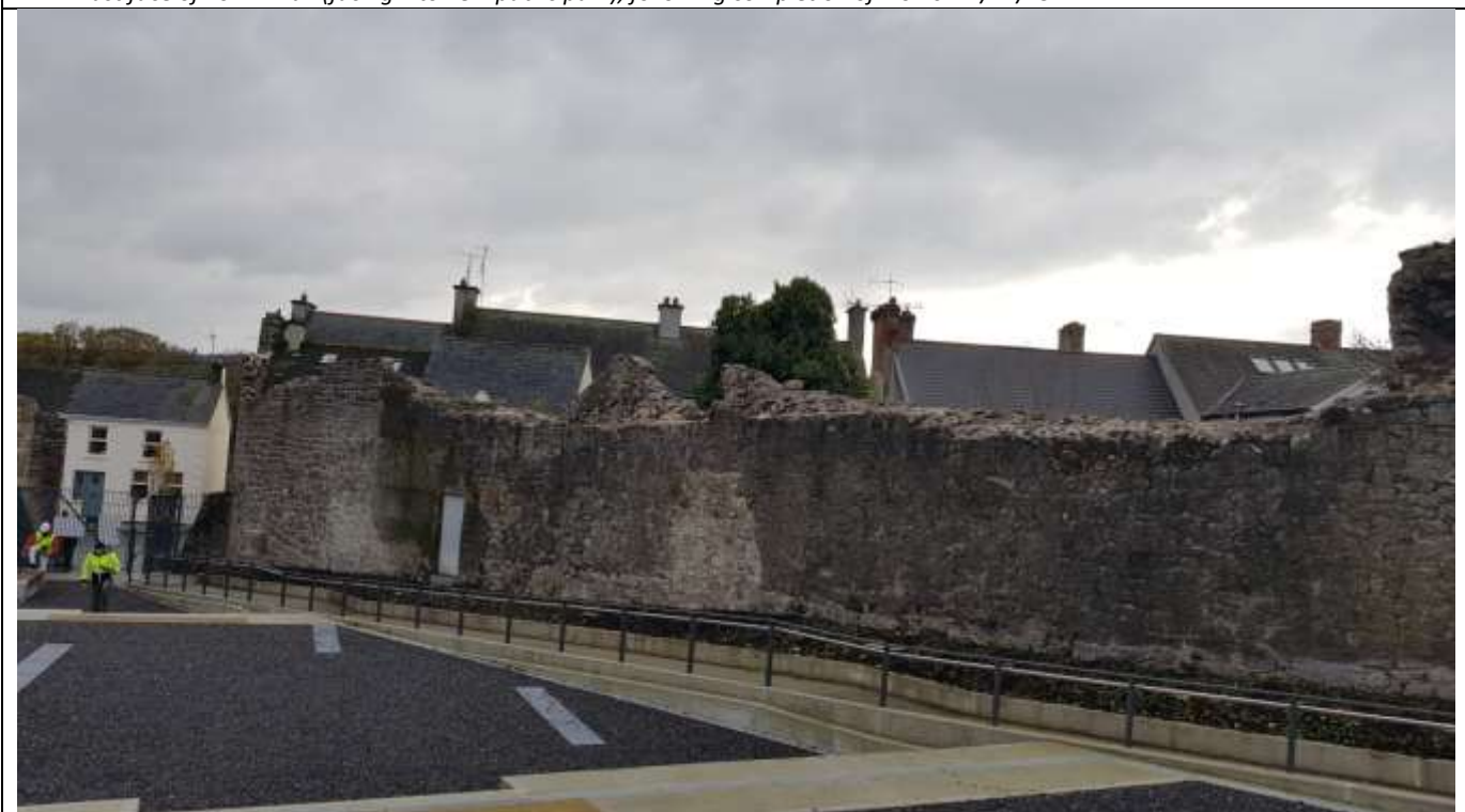
iv. Southern part of wall, with consolidated masonry at top of wall and reinstated stone rubble infill within earlier opening – 7/11/19
