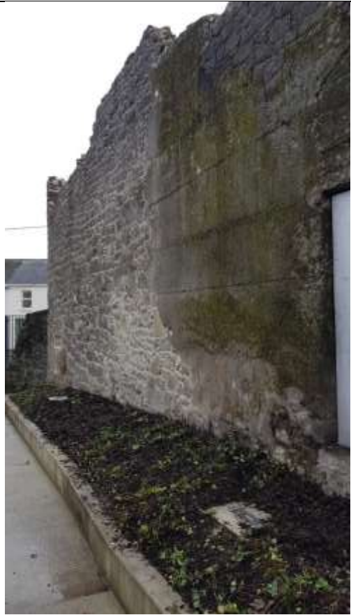
vi. Re-pointed mortar joints at southern end of wall – 7/11/19
