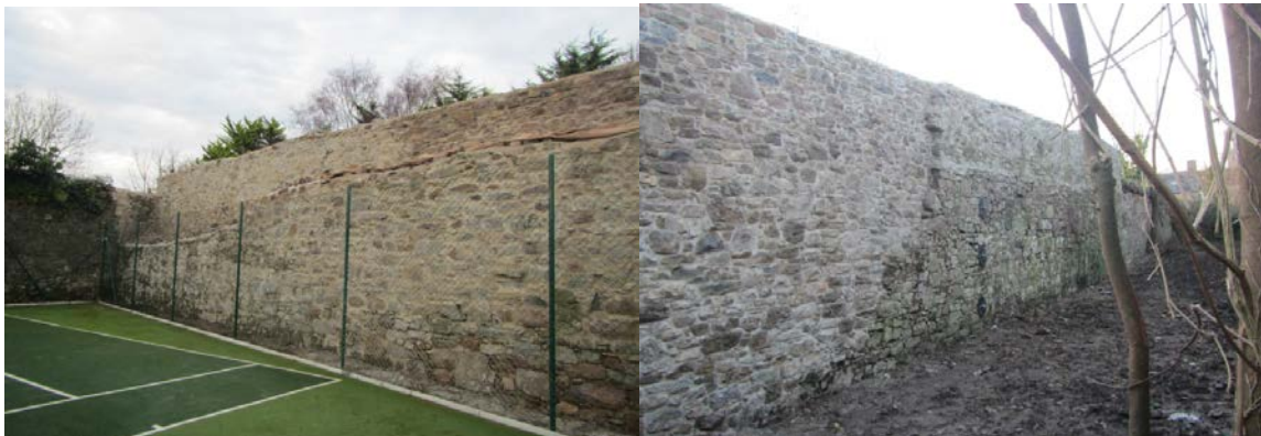
Figure 1: Works complete at Carrick on Suir
