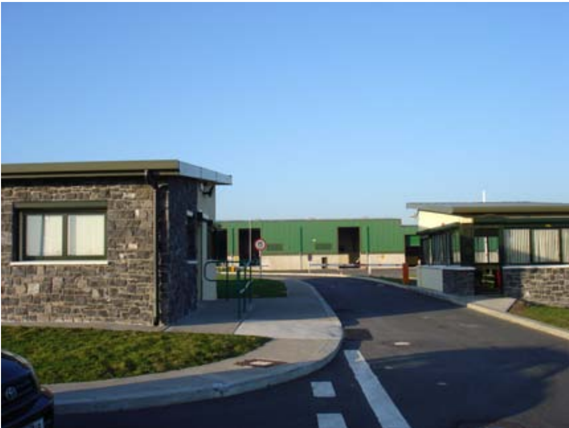
Figure 8.2: Cashel Recycling Centre and Waste Transfer Station at Wallers Lot
