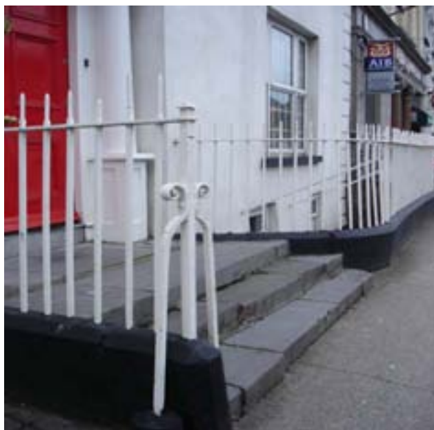
Figure 6.1: Limestone steps and wrought iron railings.
