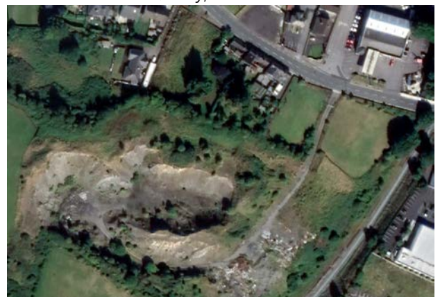
Birr Road Former Quarry, Aerial View
