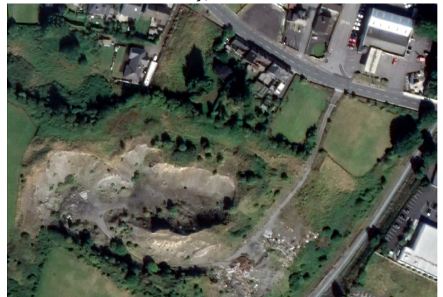
Birr Road Former Quarry, Aerial View
