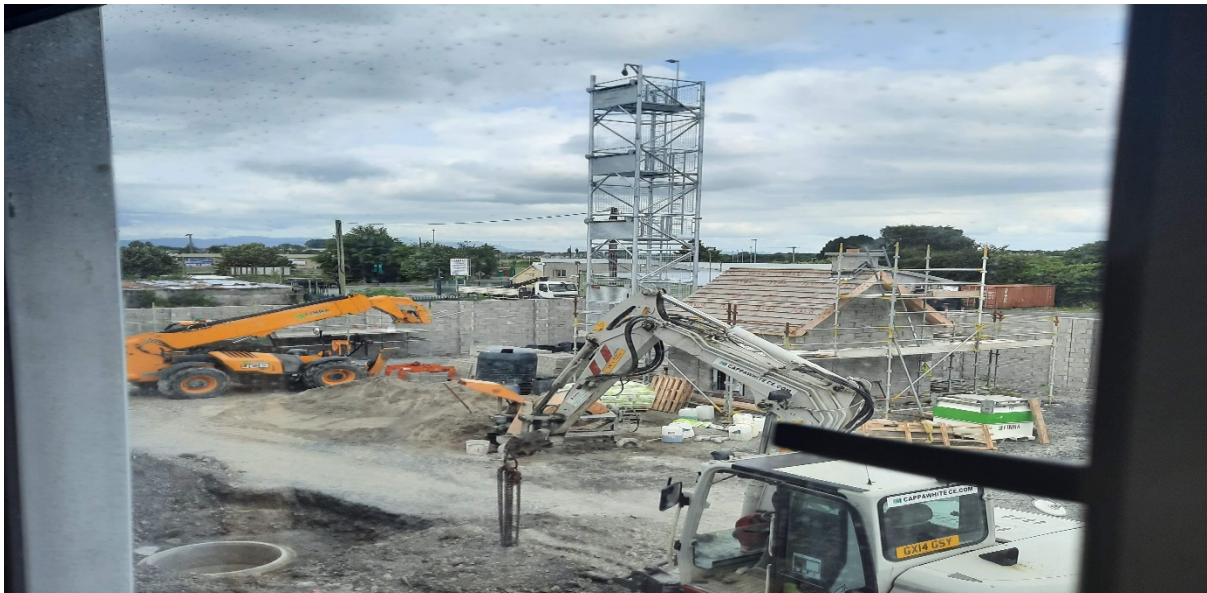
New Cashel Fire Station
