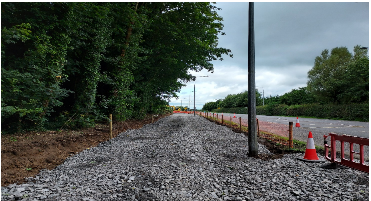
R445 Roscrea – in progress
