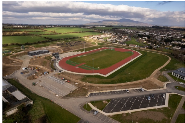
Clonmel Regional Sports Hub Completed
