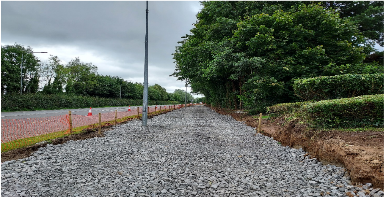
R445 Roscrea – in progress
