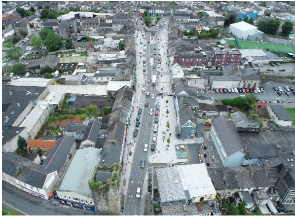
Liberty Square Phase 1 Completed
