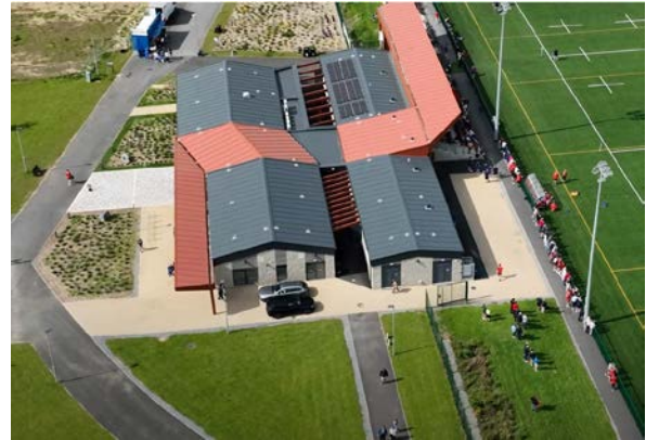
Fethard Town Park Completed
