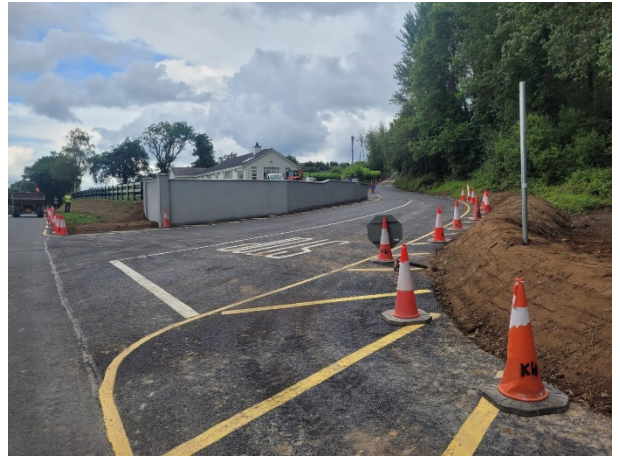
Loughtea Junction Safety Scheme
