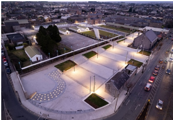
Kickham Barracks Plaza Completed
