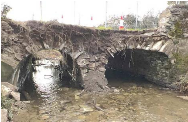
Gullett Bridge - Before
