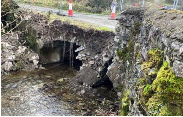
Gullett Bridge - Before
