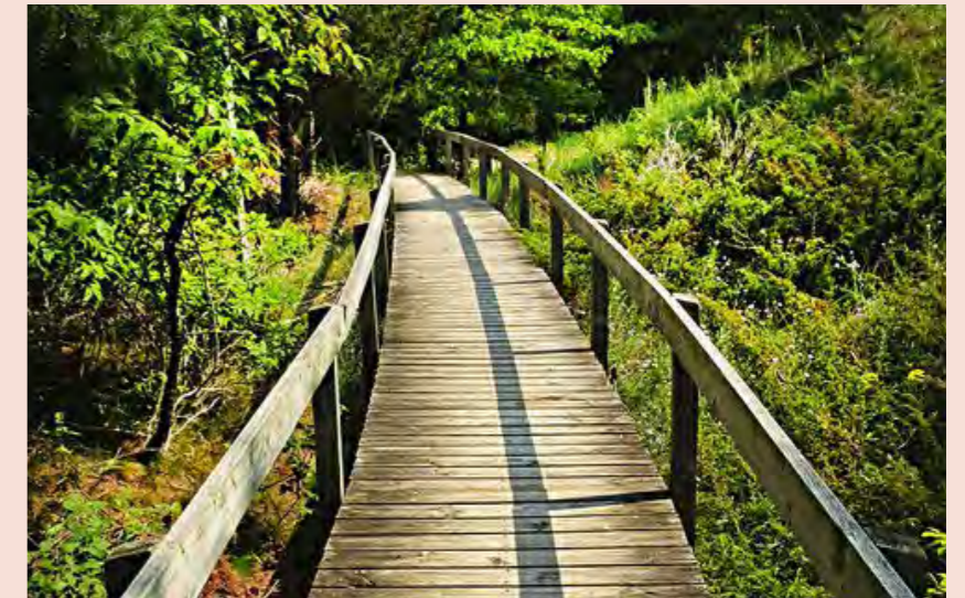
Wooden bridge connecting to Ball Alley site
