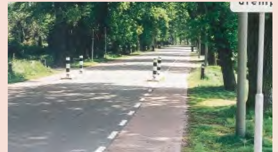
Road with demarcated shared walkway/ cycle lane as proposed for Custom Gap Road
