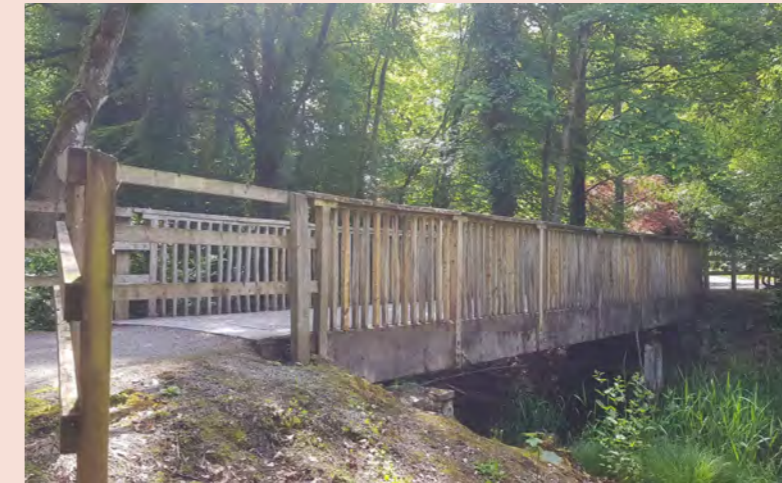
Bridge across River
