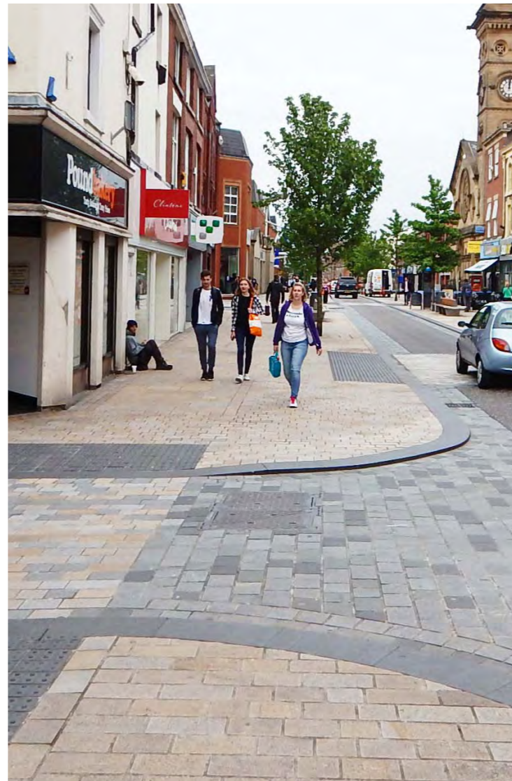
Raised pedestrian crossing
