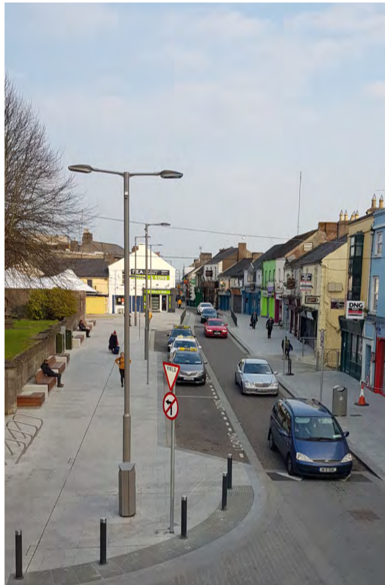
Buildout to create pedestrian zone
