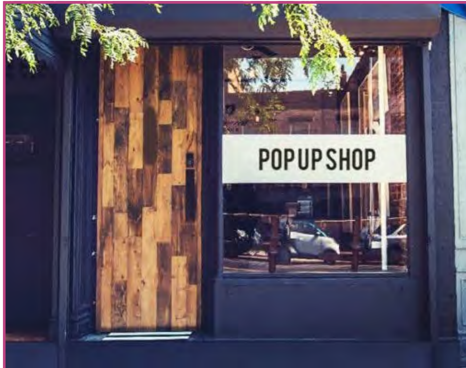
Pop-up uses for vacant buildings
