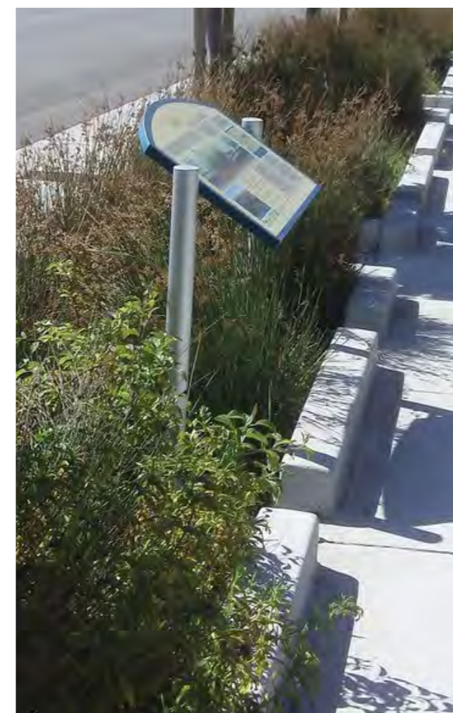
Rain gardens & SuDS
