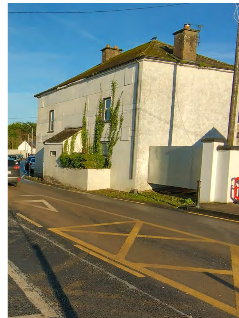
Disconnect in footpath
