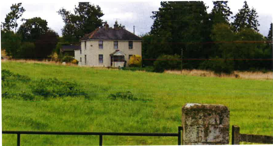
Figure 4 Dwelling on site
