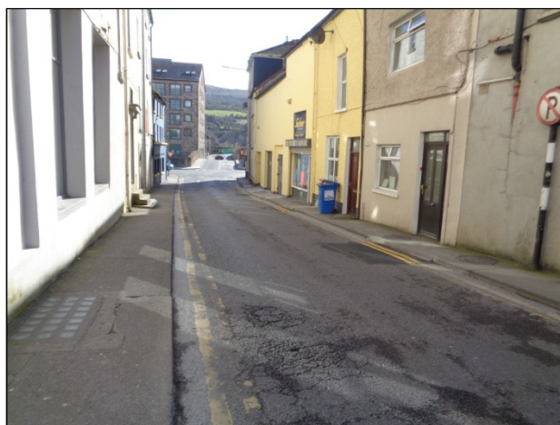
Pl. 6 Looking South along Bridge St.
