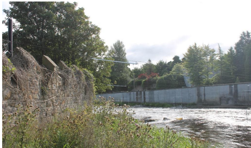
Figure 19: River wall to south of Suir Island (ref:0904.01-03), September 2017
