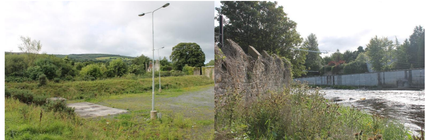
Figure 3: Flood defence berm (left); flood defence wall (right)
