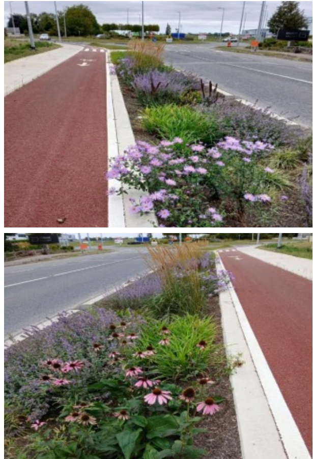
Figure 53: Rain gardens installed on the Cashel Road Active Travel Scheme
