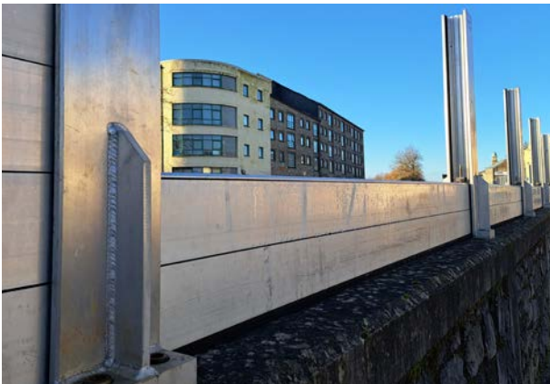
Figure 51: Flood Defences erected along the Quays in Clonmel in response to flood risk
