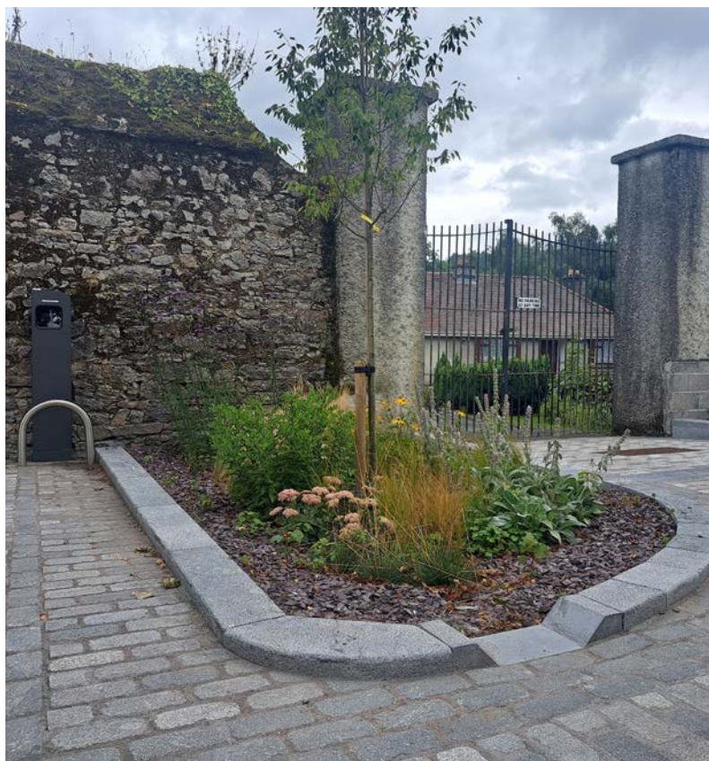
Figure 55: Rain Garden at Ormond Castle Park, Carrick on Suir
