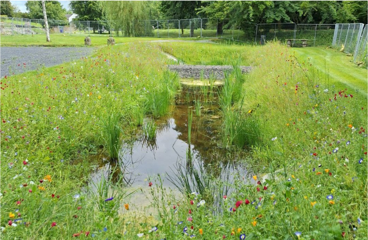
Figure 1: Nature Based Solutions to surface water management from car park in Tipperary
