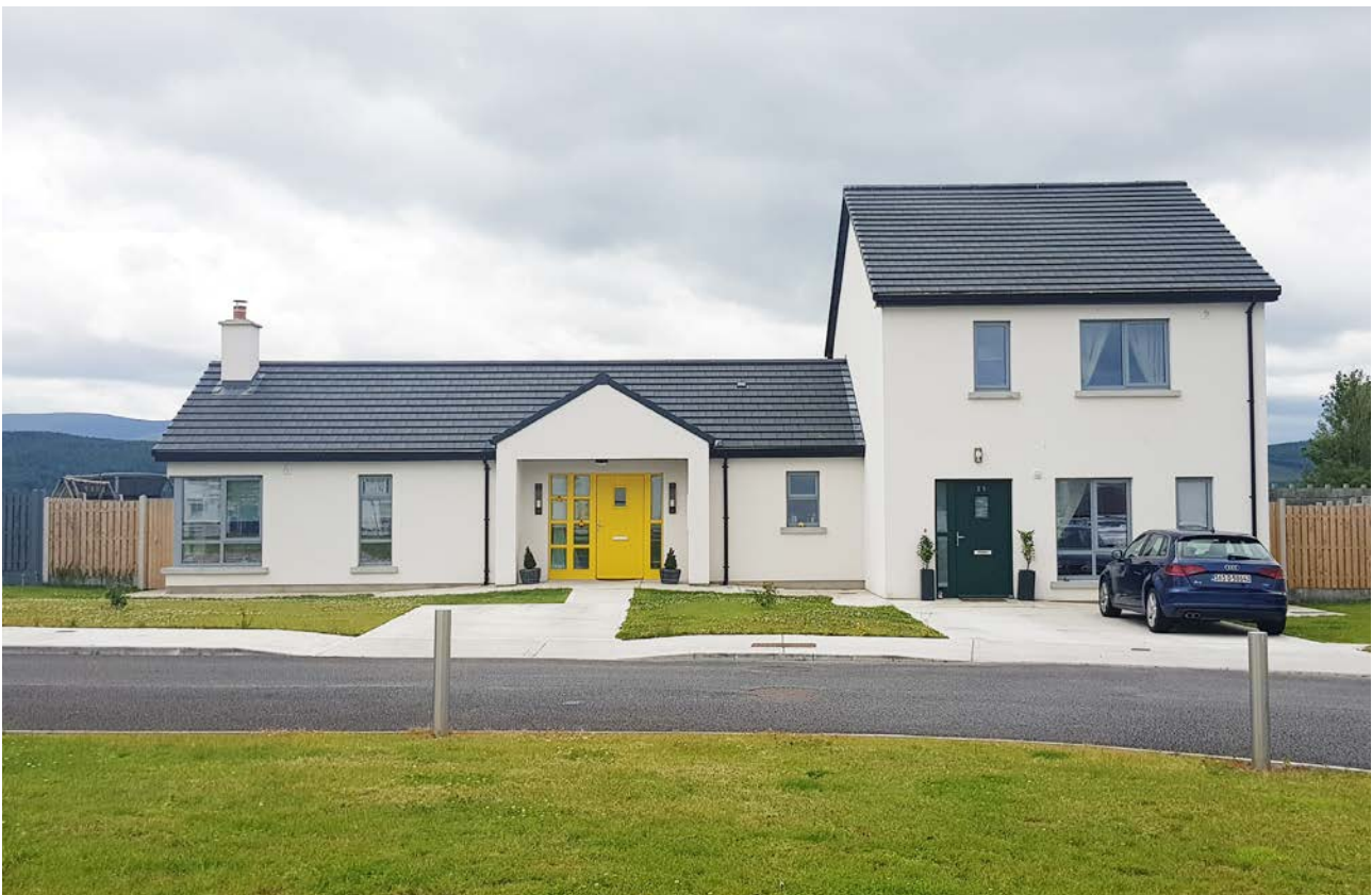
Figure 72: New Homes in Tipperary Town
