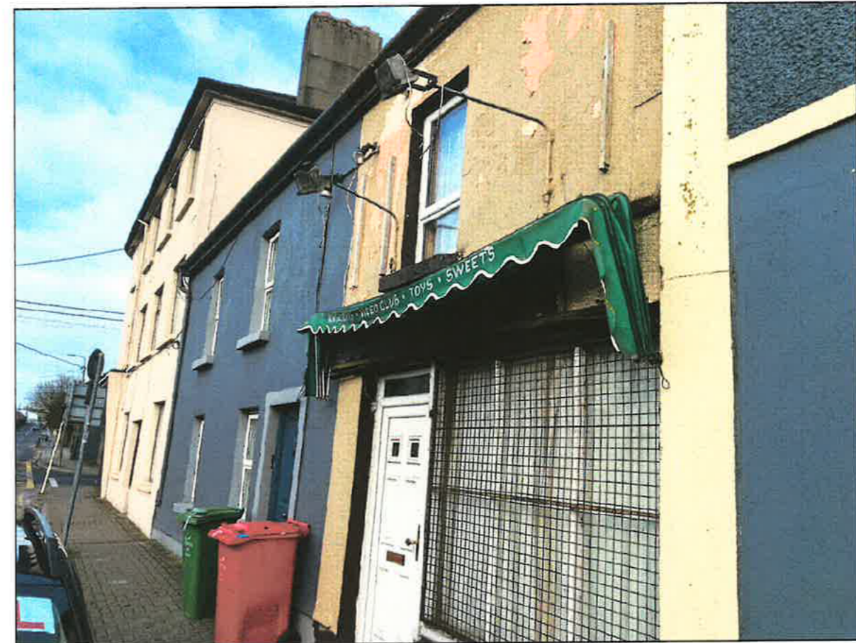
VIEW OF EXISTING SHOPFRONT
