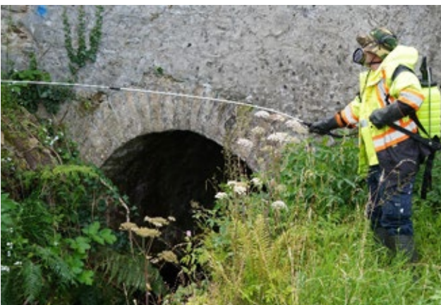
Treatment underway by contractors engaged under the Farming for Water EIP project.
