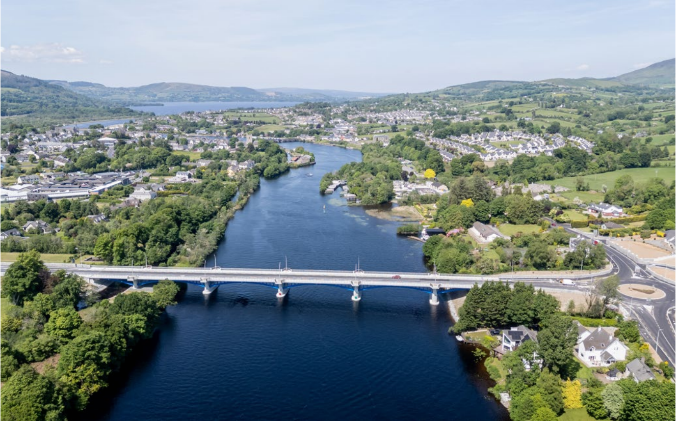
Ballina/Killaloe Shannon Bridge Crossing – Brian Ború Bridge – works complete 2025
