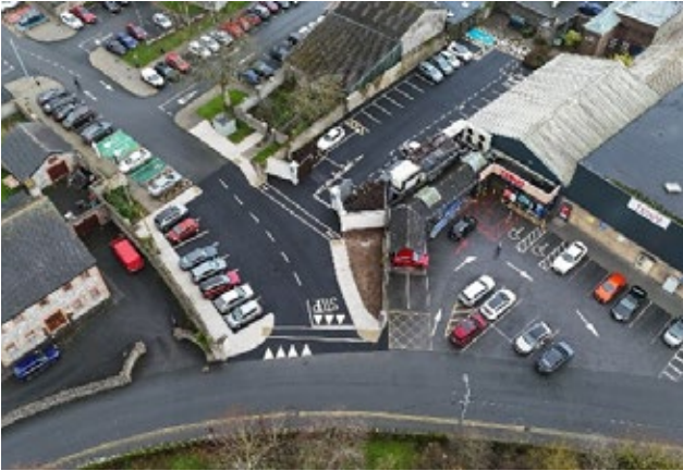
New carpark extension at Slievenamon Road carpark, which now allows access to Emmet Street.
