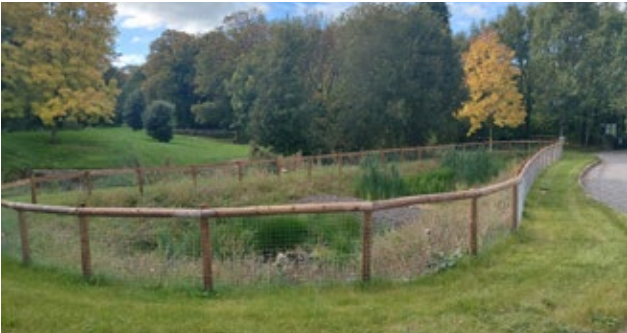
N65 Carrigahorig Village Pavement Improvement Scheme Advance Works – Attenuation Pond Completed 2025
