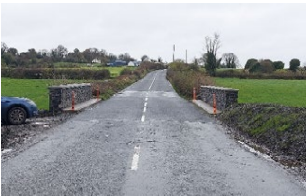
Replacement of collapsed culvert on the R438 at Graigue
