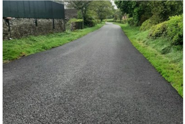
Rathdrum L-7201 Road improvement Works
