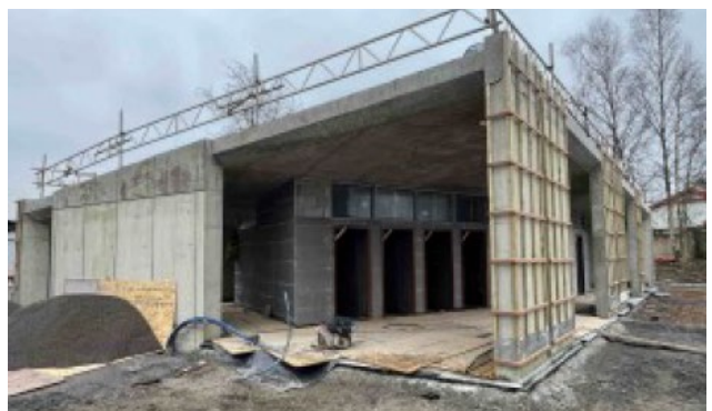
Construction of Water Sports Facility at Dromineer
