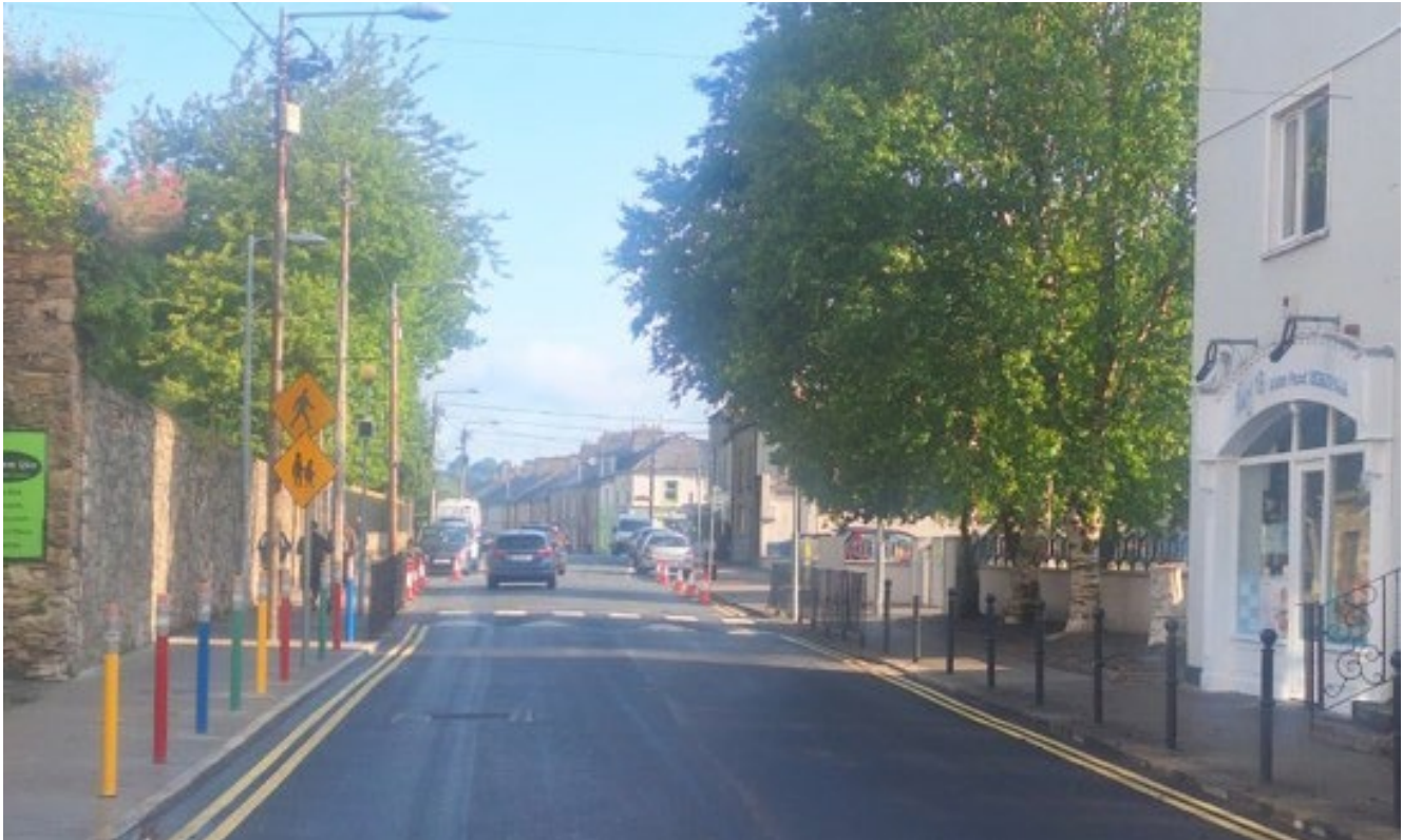
Mary St – New footpaths, road surface and pencil bollards
