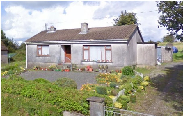
Void property before works
