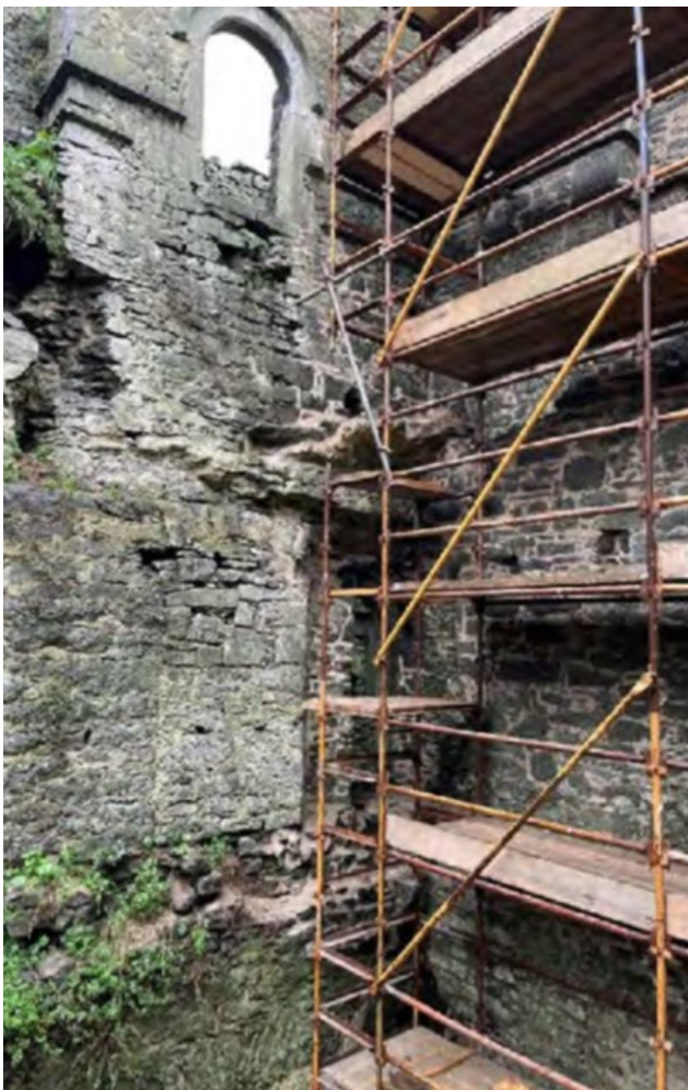
Repointing at Northwest corner Loughmore Castle
