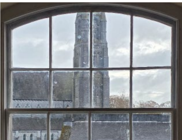
Window Conservation work completed at Nenagh Governor's House
