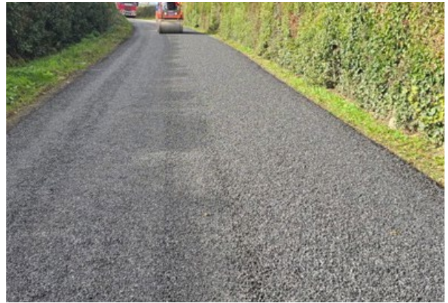
Ballyvaughan L-2507 Road Improvement Works
