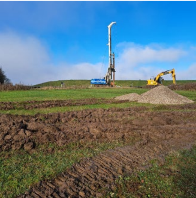
Ballaghveny Landfill – Phase 1 Capping Project drilling of new monitoring wells November 2025
