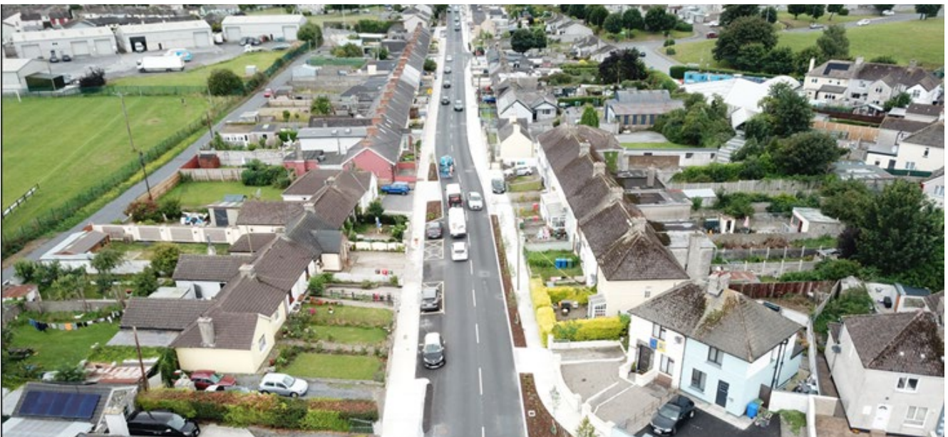
N74 Fr. Mathew Street, Tipperary Town Road Improvement Scheme – works substantially complete 2025
