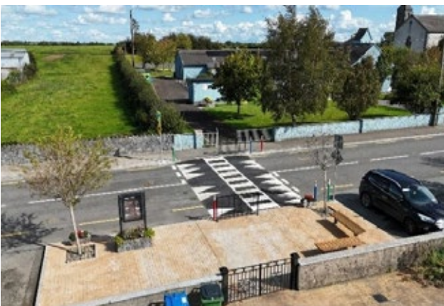
Speed ramps and pedestrian crossing installed at Drom, N.S.
