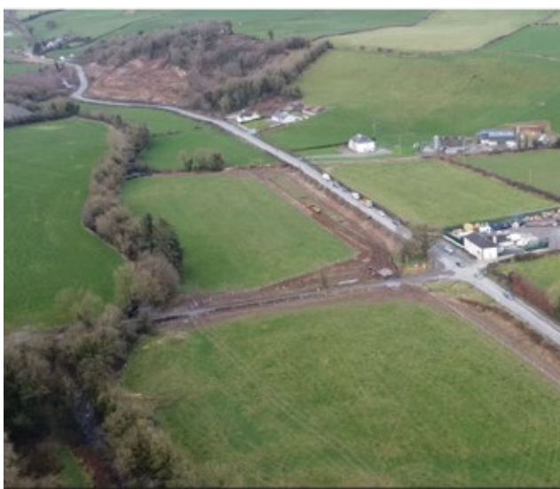
R498 Road Re-Alignment at Latteragh Bends Site Clearance and Fencing Works
