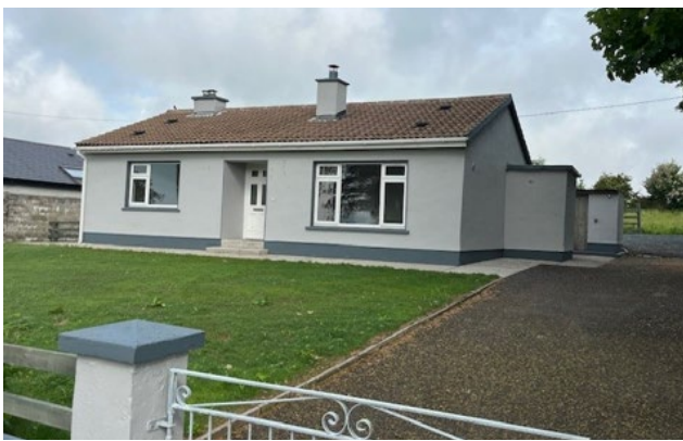
Property after completion of works
