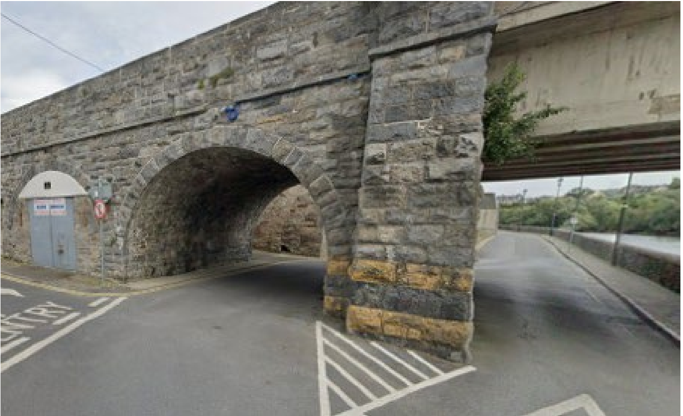
Dillon Bridge Arches
