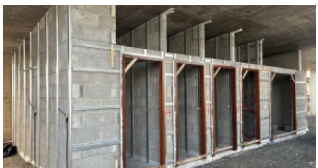
Construction of Water Sports Facility at Dromineer
