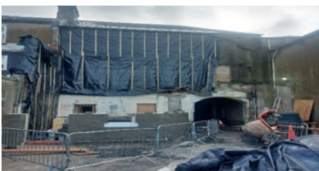
Figure P10 Market House Enabling Works, Cahir
