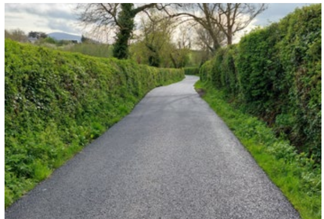
Orchardstown East L-7204-0 Road improvement works
