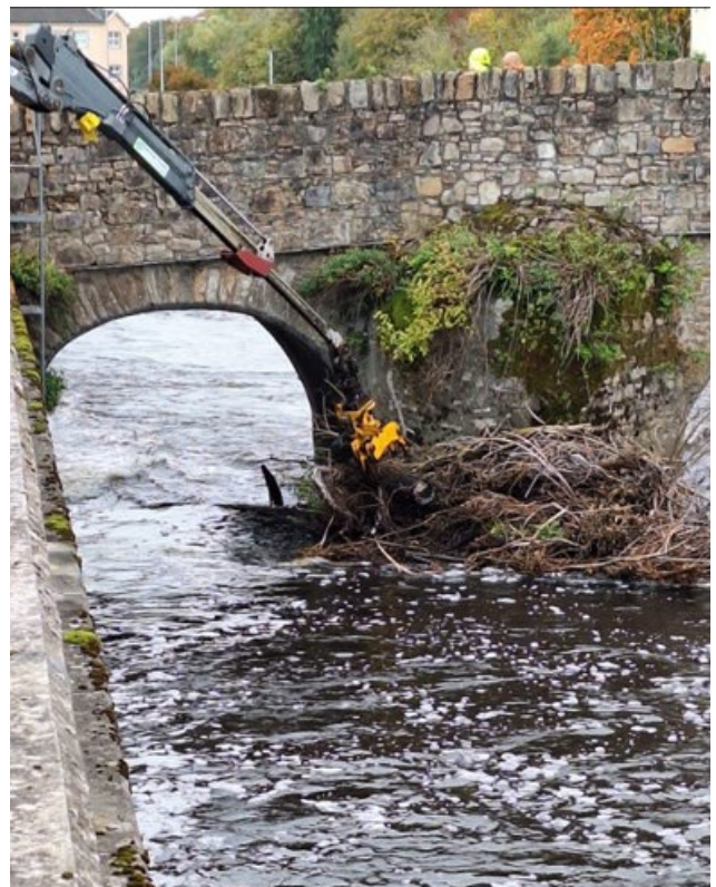
Removing vegetation from the Old Bridge
