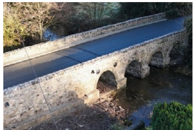
Refurbishment Works on Farney Bridge, Holycross.
