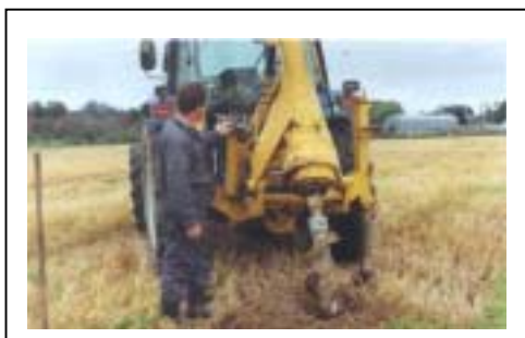
Plate 7: Tractor-mounted auger Photo: J. Keohane)
