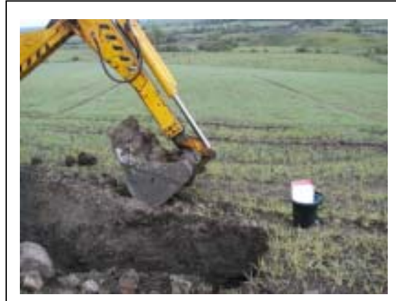
Plate 9: Mechanical Digger & trial hole (Photo: D. Kelly)
